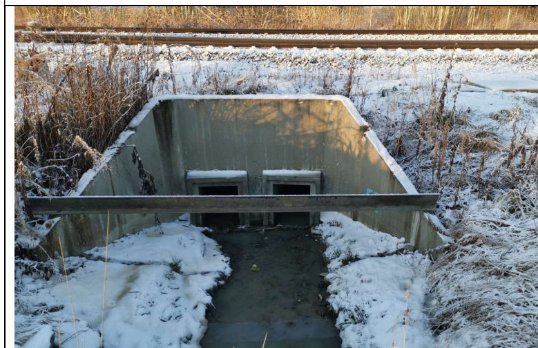
Kulvert under Dovrebanen for Lersbekken (Norconsult 2019).
